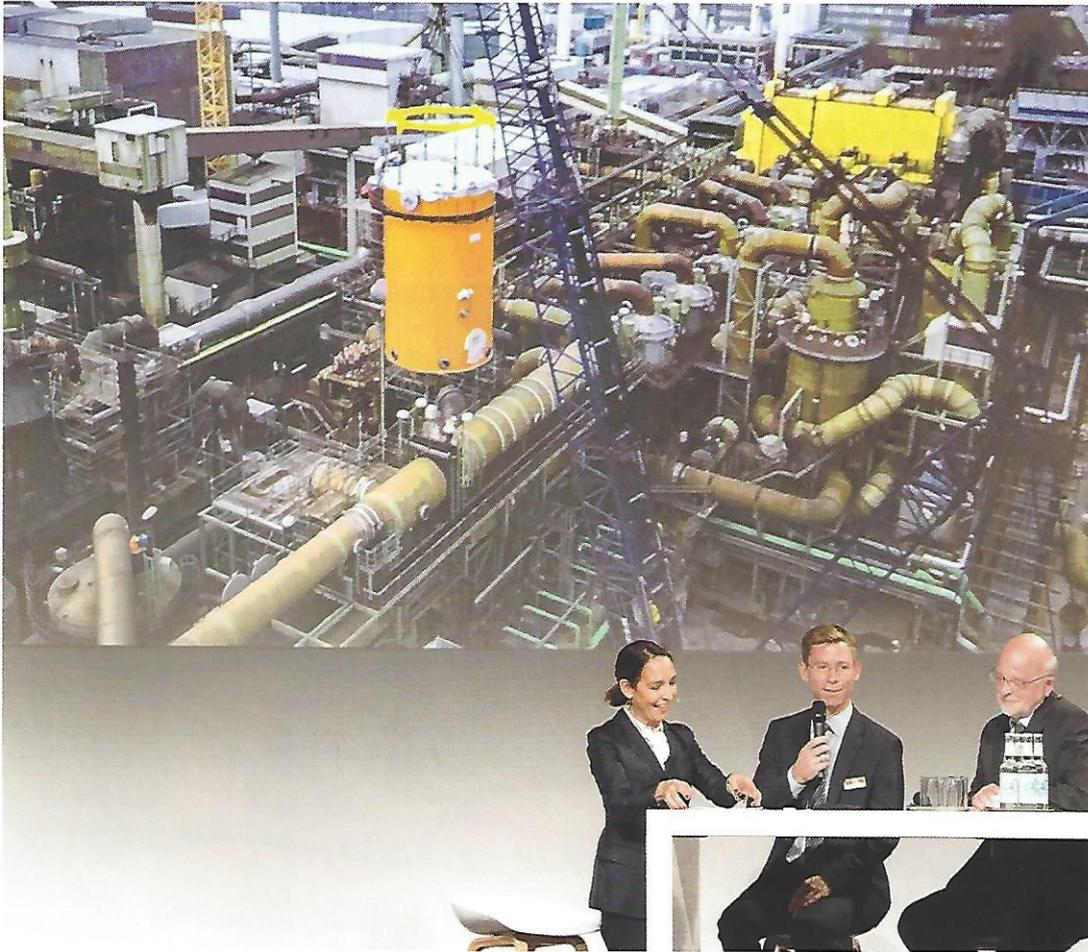
The sulfuric acid is formed in the intermediate absorber (orange silo) of the acid plant. Aurubis extracts the CO<sub>2</sub>-free heat released during this process and has been using it to supply a new district of Hamburg since the fall of 2018. The picture shows TV presenter Andrea Thilo (l.), Christian Hein of Aurubis, and Dr. Martin Schüle of enercity at the opening of the multi-award-winning project
